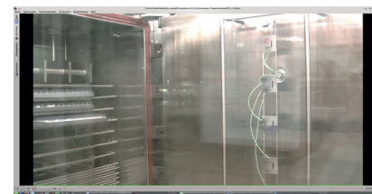
Fig. 16: TEMPRIS antenna installation in the freeze dryer.
